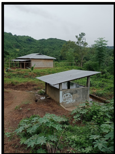
Figure 5: The community water tank in Nobo Gurubari Village
